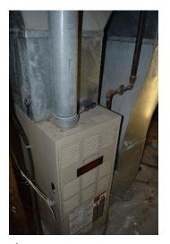
Air Conditioning unit is a Coleman model 7036-811 Serial Number is 048505624 3 ton unit manfuctured in April 1985.
