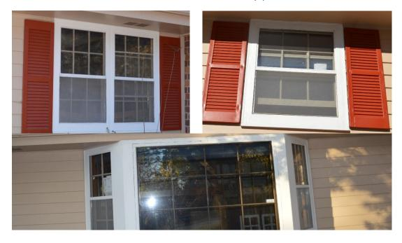
Exterior; Freshly painted wood siding. No missing pieces found. House looks very good. Windows on the front and east side have nonfunctioning fiberglass shutters that have been painted a contrasting color. Garage doors in original picture have not been painted. They are slated to be replaced (white).
