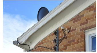
Gutters and down spouts: Despite the eves being in a condition of needing repair the gutters are is surprising good condition. No dents, separations or evidence of leaking found. Gutters in front of house are piped
