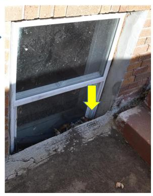
point out that this window is in the side walk to the side door of the home. If a window well is installed here it will need to be cut into the side walk. Or side walk removed and a new walk poured in after window well is installed. Window well will need a flush mount grill on top to prevent someone from falling into well.
