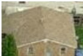
Roof: Fiberglass singles in serviceable condition with no issues found. Roof reported to be 15 years old. No torn shingles or depressions noted in roof.
